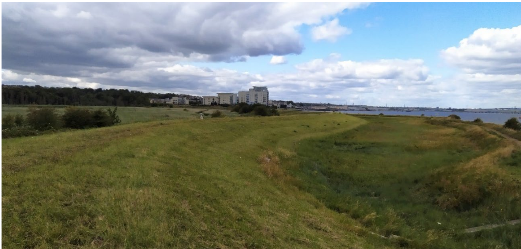
Figure 17.13: The London Resort Kent Project Site existing formal flood defence berm at Black Duck Marsh (photograph taken during site visit 28/07/20, looking southwest).
